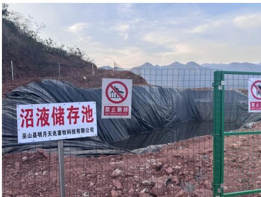
灌溉区沼液暂存池 (3000m 3 )
